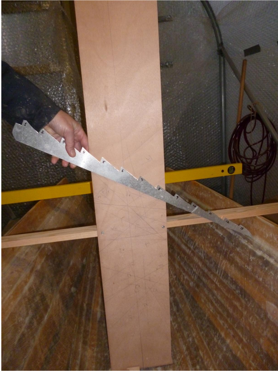
Figure 19: Measuring Transom Profile Below Knuckle
